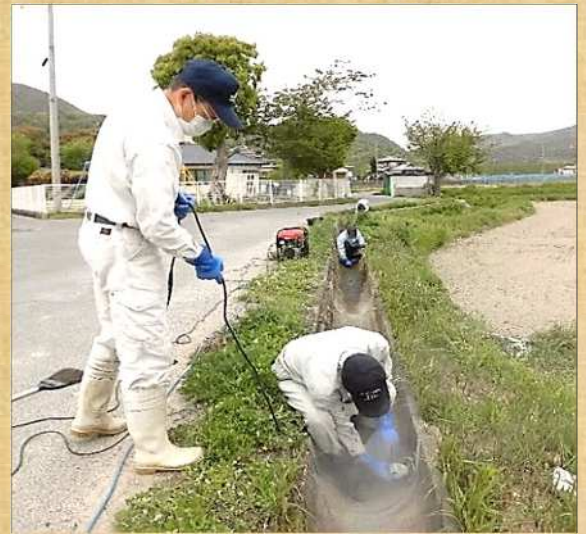
④水路の軽微な補修
